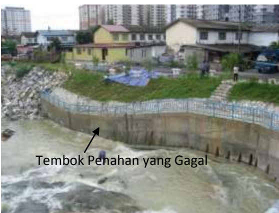
A. Before Project
