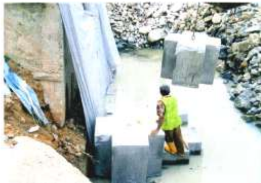
II. Lifting & Placing at site
