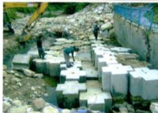
IV. Completed VIP LINER
