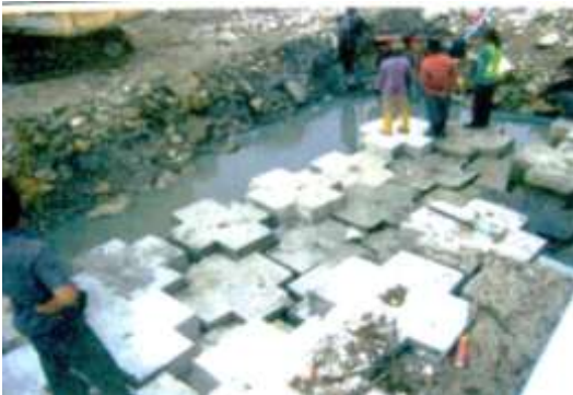
III. Placing and Arranging BLOK
