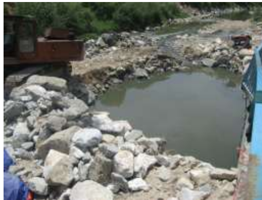
Figure 7: Exampe of site Preparation Prior to Placement of VIP LINER
