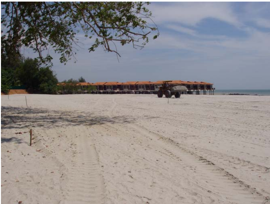
Figure 3: Beach nourishment creates additional beach space enhancing local economic potential (Port Dickson, Negeri Sembilan; November 2004)
