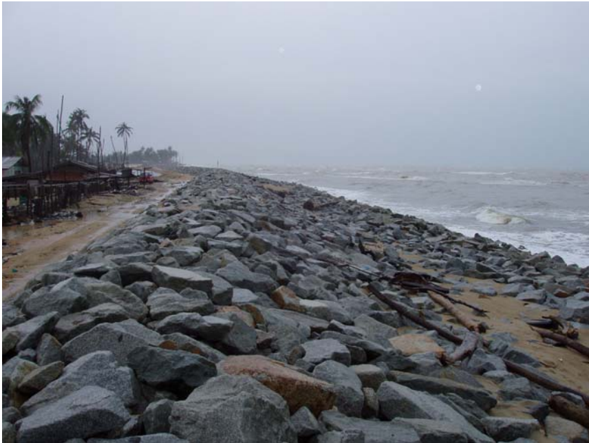
Figure 2: Rock revetments usually results in the narrowing of beaches
