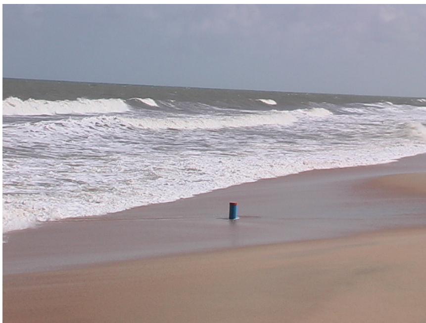
Figure 8: Pressure Equalisation Module pipe at Teluk Cempedak beach
