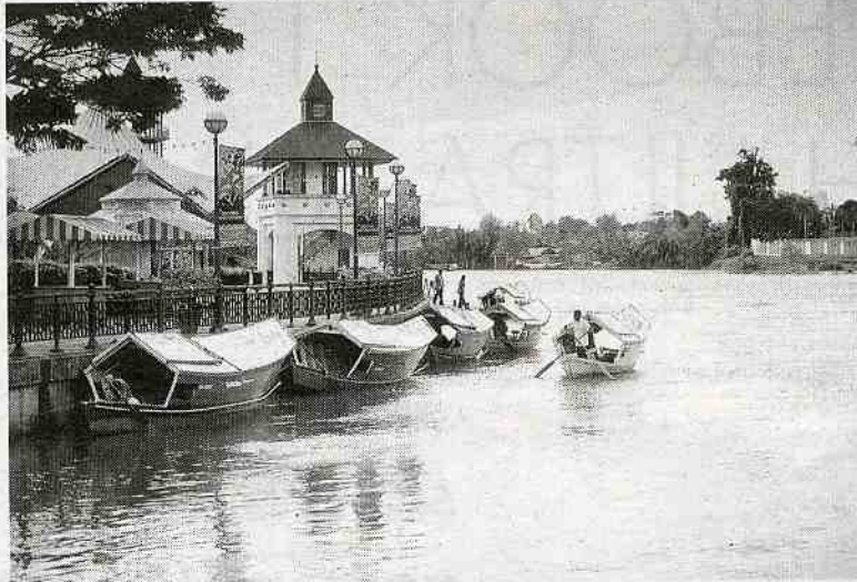
River of life: The Kuching Waterfront extension project involves massive land reclamation along the Sarawak River.
